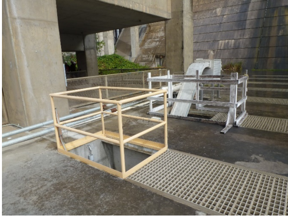
Figure 1. JDA North Fish Ladder lamprey passage structure.
